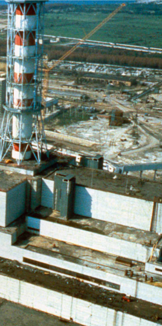
The 245-tonne steel dome is placed on Hinkley Point C's first reactor building during construction in 2023
